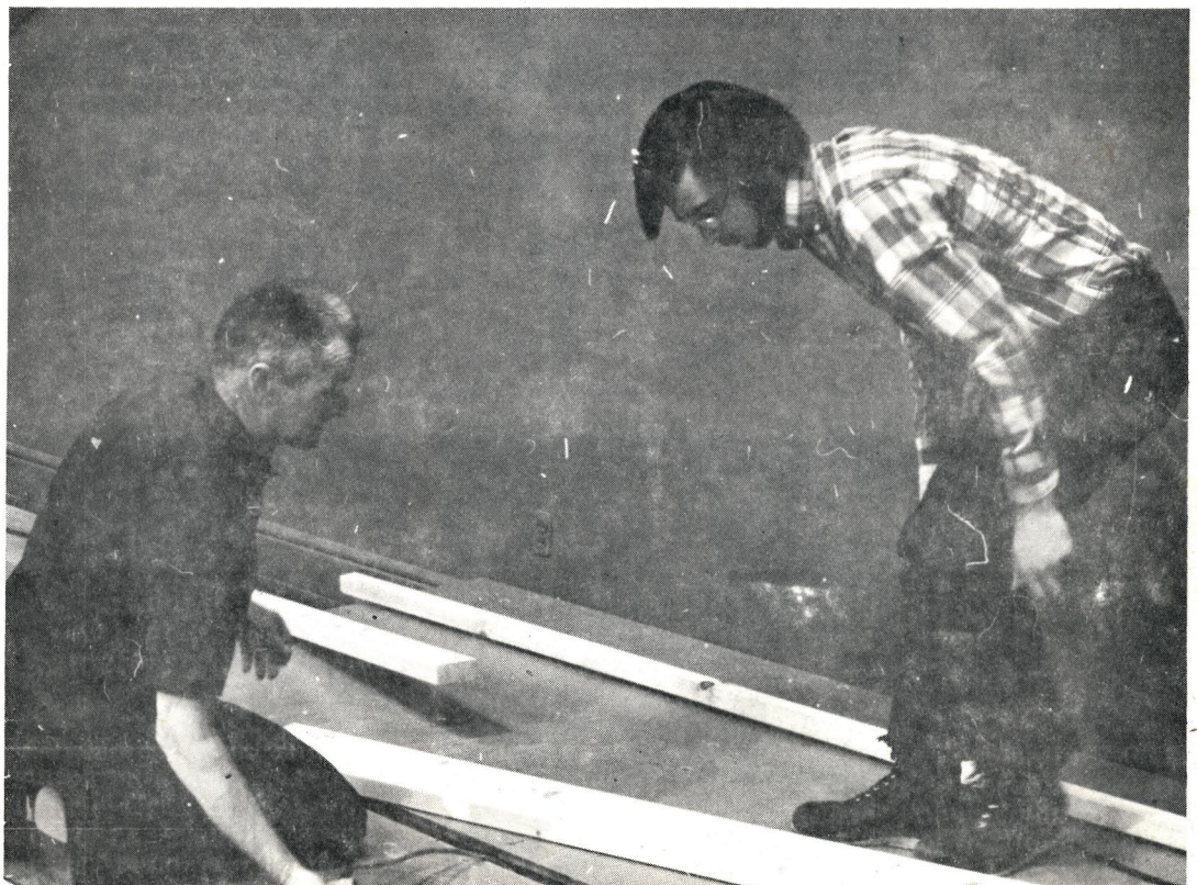
Set crews at work.
